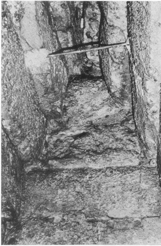
1. The roof of the burial chamber in the Meidum pyramid. The blocks are well filled, but have remained undressed
